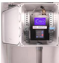
Model F-20: Measures 20 electrodes from one or two probes
